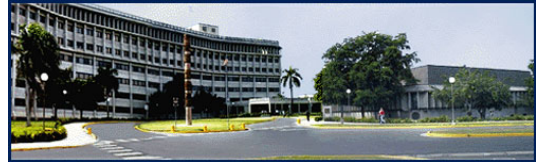
The Clemente Ruiz Nazario United States Courthouse and Federico Degetau Federal Building are 35-year old interconnected structures which are currently under renovation. Photo: www.gsa.gov
